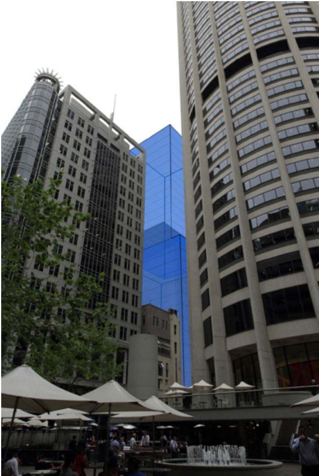
Figure 13 Proposed envelope as viewed from the lower plaza area of Australia Square.
