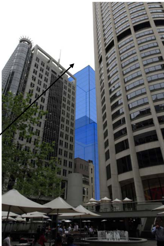
Figure 21 Comparison between DCP permissible and proposed envelopes, views from lower plaza of Australia Square.
